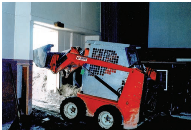
Above: Inside Floor.... The auditorium flooring was replaced removed and concreted in 2005.
