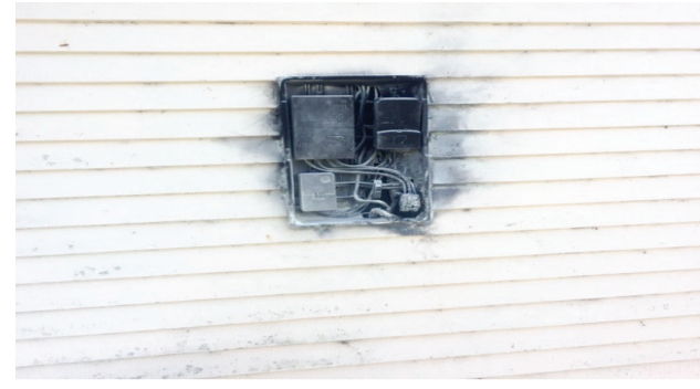
The faulty powerbox.
