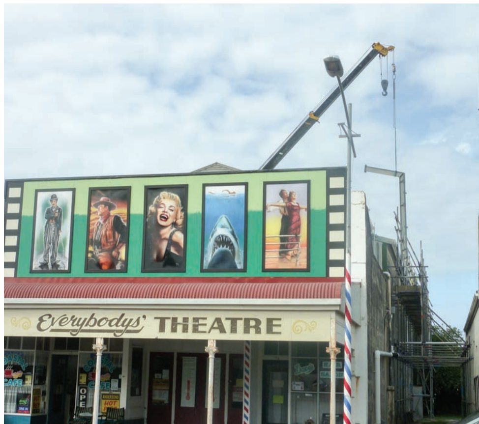
Above: Taken in 2013 when the theatre underwent structural strengthening.
